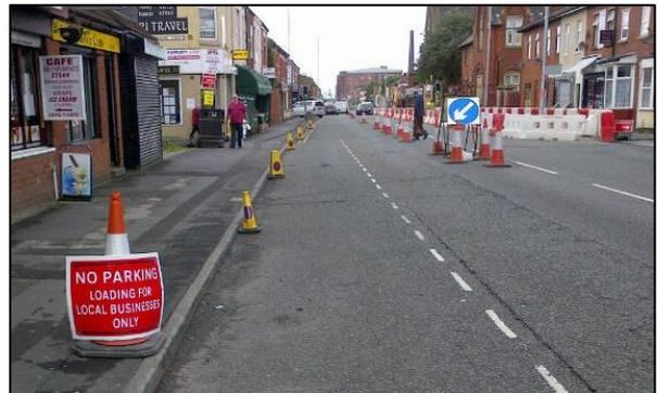
The new pavements are constructed using robust granite flags, however they are not indestructible and so we urge drivers not to park on the paving flags as it may cause them to crack or sink, as well as obstruct pedestrians from safely walking along the pavement.
